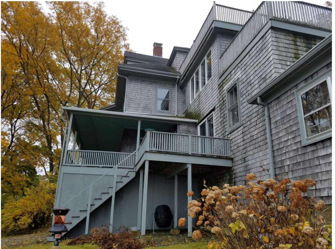
Existing Dwelling from Rear Yard
