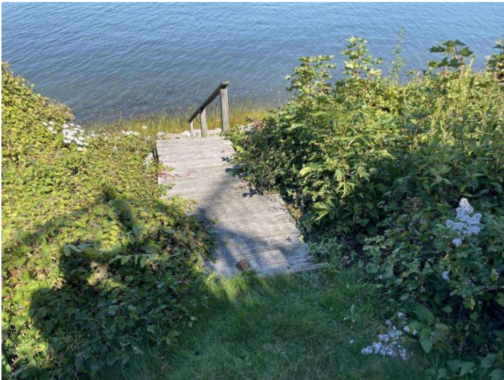
Photograph #6 – View of the existing stairway.
