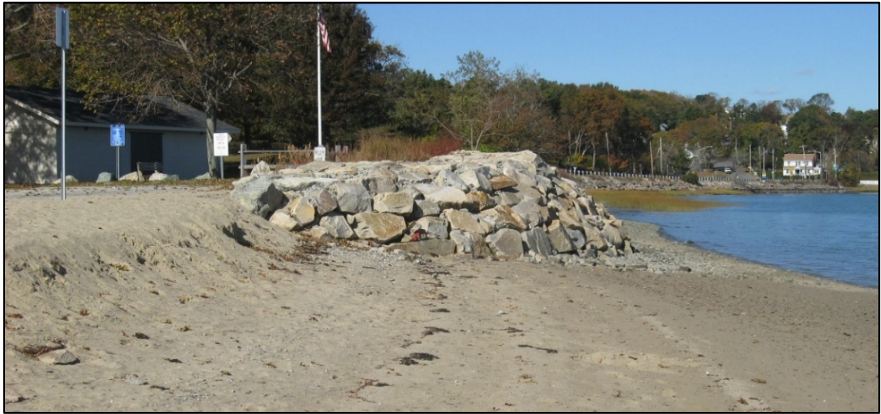
Figure 4: 2014 Reconstructed Western Revetment (Facing Northwest)
