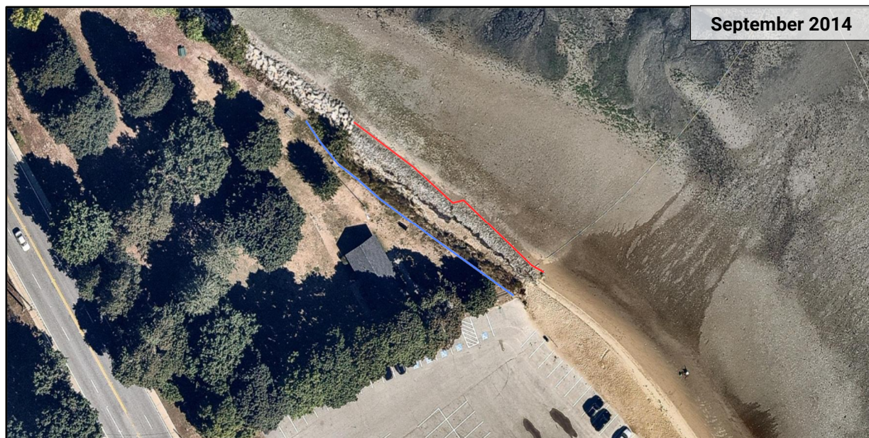
Figure 6: Shoreline position aerial photography in 2014. The red line indicates the position of the revetment toe in 2014, and the blue line represents the location of the fence line along the bank crest in 2014.
