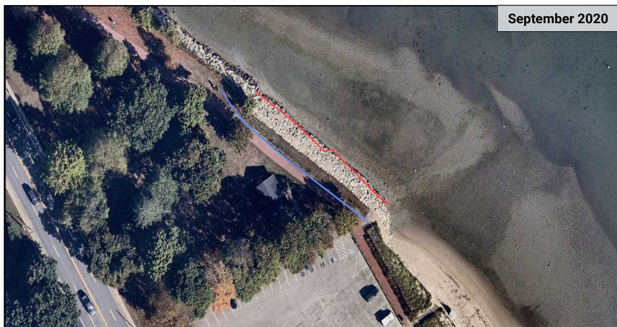
Figure 7: Shoreline position aerial photography in 2020. The red line indicates the position of the revetment toe in 2014, and the blue line represents the location of the fence line along the bank crest in 2014.
