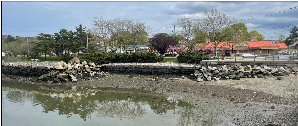
Figure 14: Existing shoreline armoring along P.O.W./M.I.A. Memorial Park
