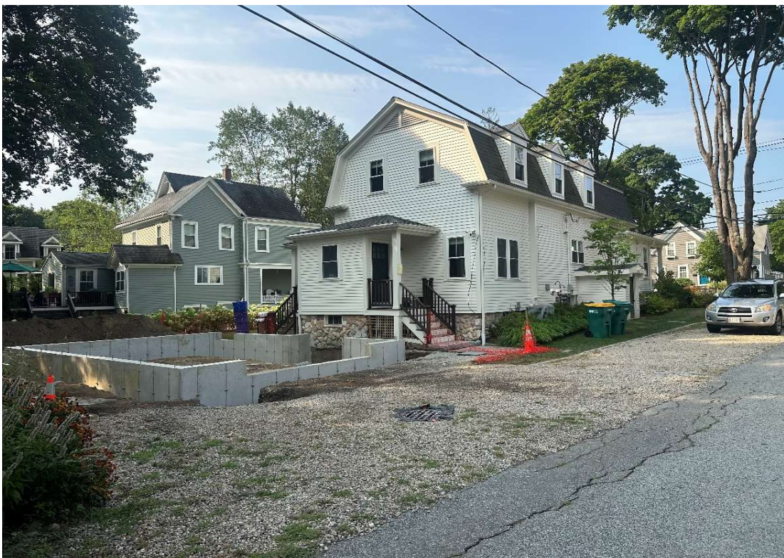
40 Hersey Street - Addition or Garage Under Construction - 42 Hersey in Background
