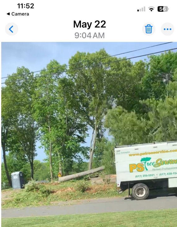
22 May tree removal photo of southern line
