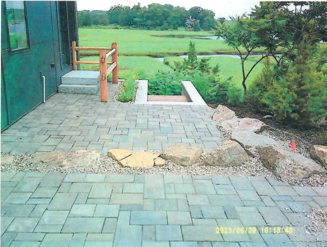
Photograph #1- View from the edge of the paver driveway towards the paver patio and stairway.
