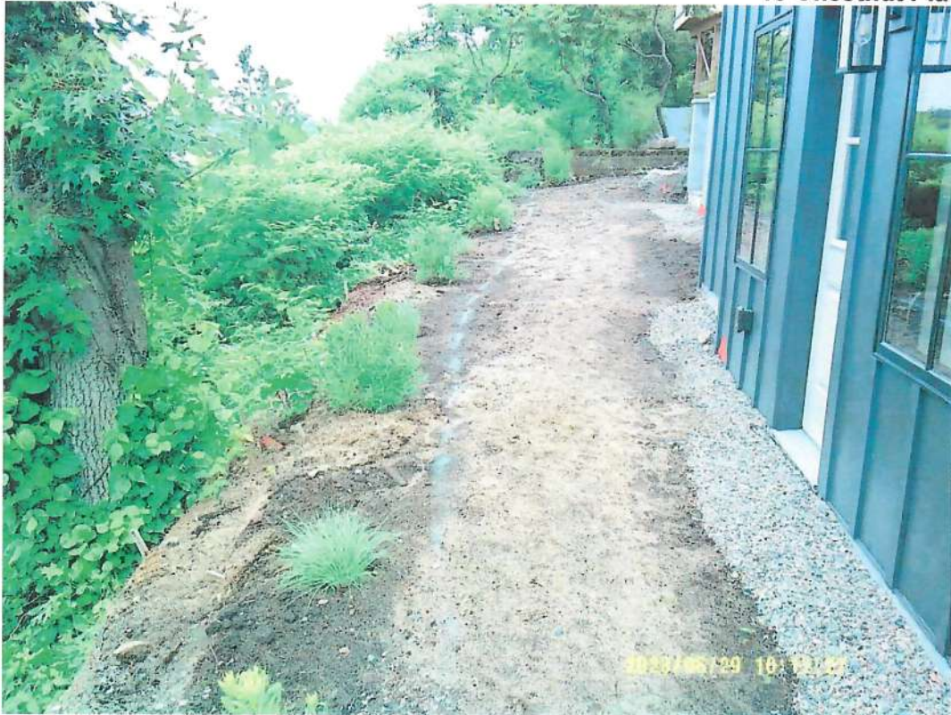
Photograph #3- View along the base of the house facing the Coastal Bank. Notice mitigation plantings, gravel drip strip, etc.
