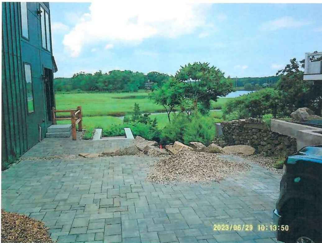
Photograph #6 - View of the paver driveway towards the paver patio, mitigation plantings, etc.
