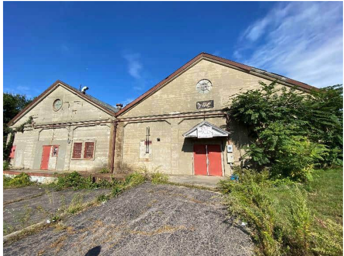
Photo 1: South end of building with access to both east (12A) and west (12B) buildings.
